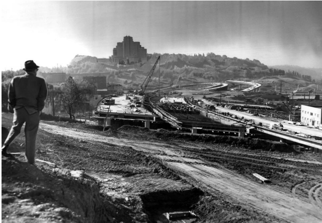
Figure 7: Man overlooking the construction of I-5 cutting through Chinatown
